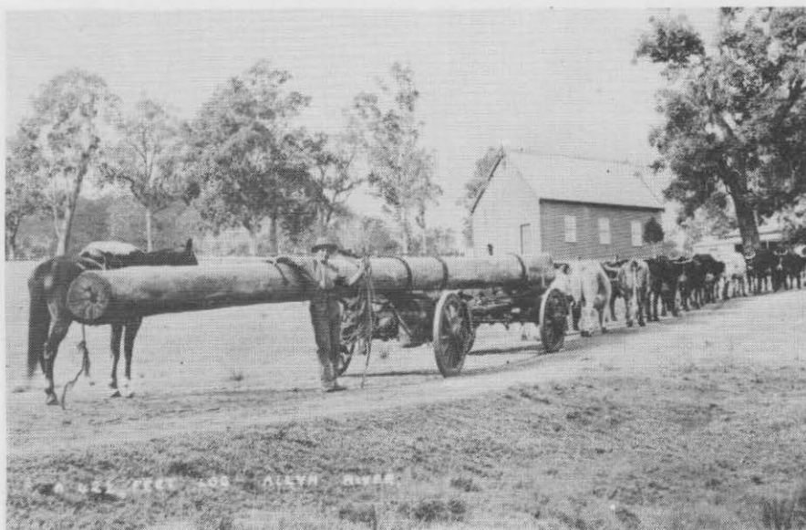
Logging in the 1920's - a 42' log on a bullock team in front of Eccleston Congregational Church. Most of the logs came from the Allyn River. Hancocks had a sawmill some miles up the river, and Norman Joliffe had a mill between Eccleston and Allynbrook.
