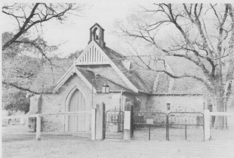
St. Mary's Anglican Church, Allynbrook
