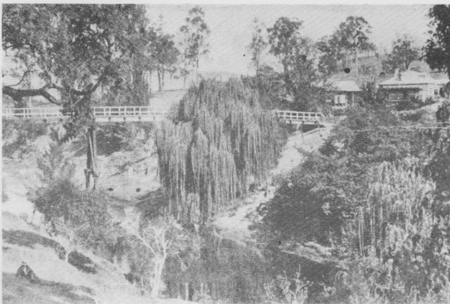
The old foot bridge on the Paterson River. The house on the right was called "Ardna-Hane" ("on the side of the hill")
